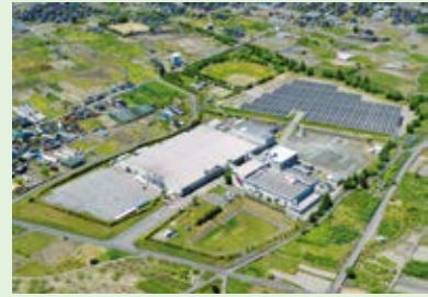
Yamanashi Factory at which Smart Factory Initiative is being advanced
