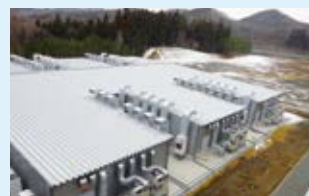
Shirakawa Data Center of Yahoo Japan Corporation and IDC Frontier Inc.
