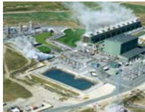
Geothermal power generation
