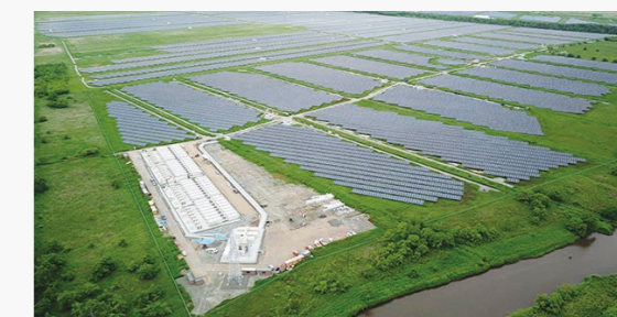
Suzuran Kushiro-cho Solar Power Plant (Hokkaido, Japan)
