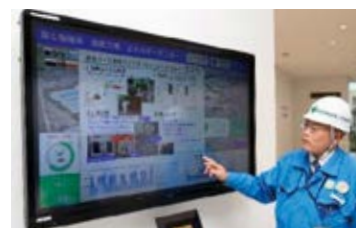
Energy usage monitoring system
