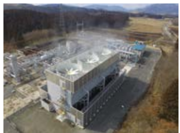
Takigami Binary Geothermal Power Station
