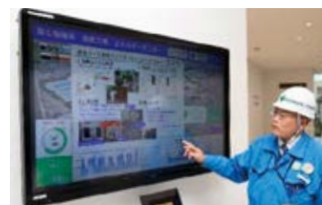
Energy usage monitoring system
