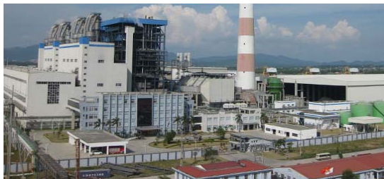
Haiphong Coal-Fired Thermal Power Station in Vietnam
