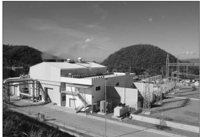
Fig.5 Panoramic view of Maibarara Geothermal Power Plant
