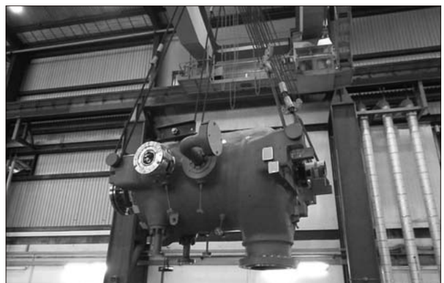
Fig.6 High-pressure turbine of Unit 12 undergoing renewal in the field
