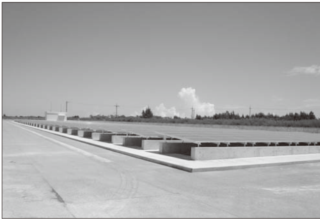
Fig.9 Overall view of system (Taramajima)
