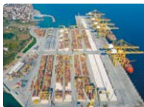
Nine crane control solution sets delivered to Asyaport Liman A.Ş., of Turkey
