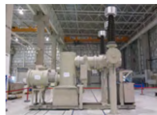
Gas-insulated switchgear
