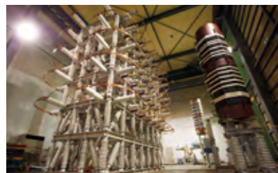
High-power testing facility (Chiba Factory)
