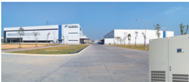
Fuji Electric Manufacturing (Thailand) Co., Ltd.
