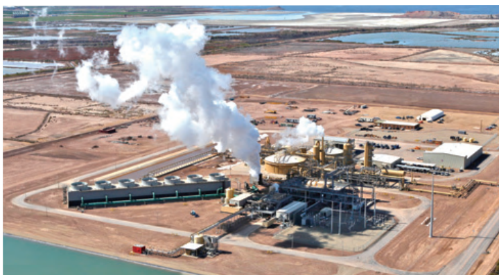
Hudson Ranch I Geothermal Power Plant (HRI): HRI and HRII each generate enough power to serve 50,000 homes in the Southwestern region of the U.S.
