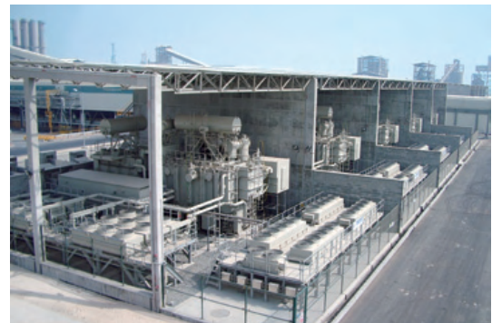
This photo at EMAL's aluminum smelting plant shows some of 12 S-Formers delivered for first-phase construction. Once six more S-Formers are delivered for the second phase, the smelter will be among the world's largest
