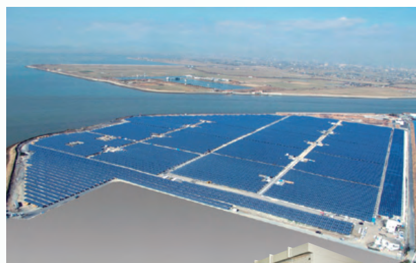
Work to expand orders and sales of solar power generation systems (Kyushu Solar Farm 7 Miyama Joint Power Station)
