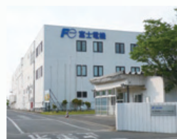
Fuji Electric acquired a subsidiary of Renesas Electronics Corporation and established Fuji Electric Tsugaru Semiconductor Co., Ltd. with a view to enhancing its production capacity for power semiconductors and dispersing risk
